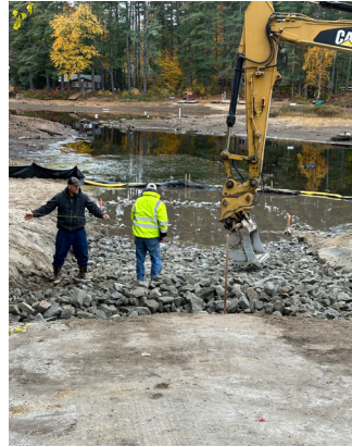
Ramp bed preparation
