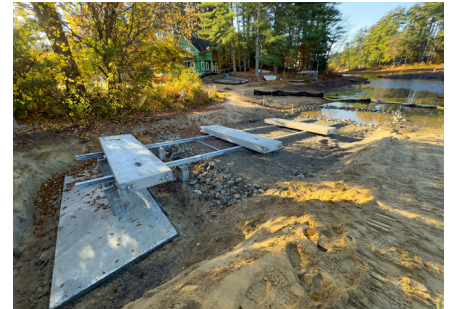
Concrete planks being affixed
