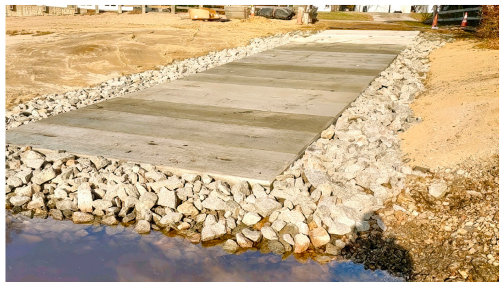
Completed Ramp, photo by Rick Blank
