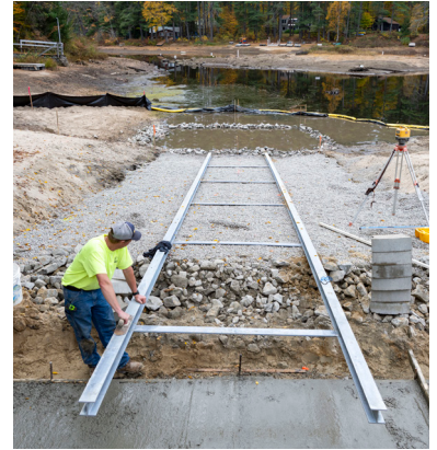
Steel I-beams being placed
